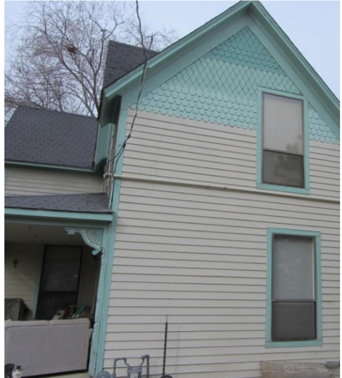
Figure 5: Main Service Entrance
